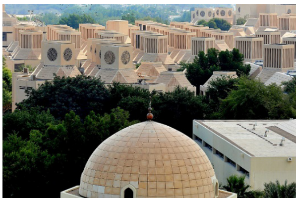
Figure 7: The Educational Technology Facility uses Wind Towers to Encourage Natural Ventilation Source: University 38 .
