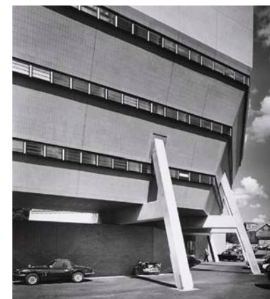
figura 17 Leicester University Engineering Building, 1959-1963 Reference number: AP140.S2.SS1.D23.P12.9
