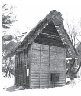
*2. Nakano Yoshimori Storage Shed.
